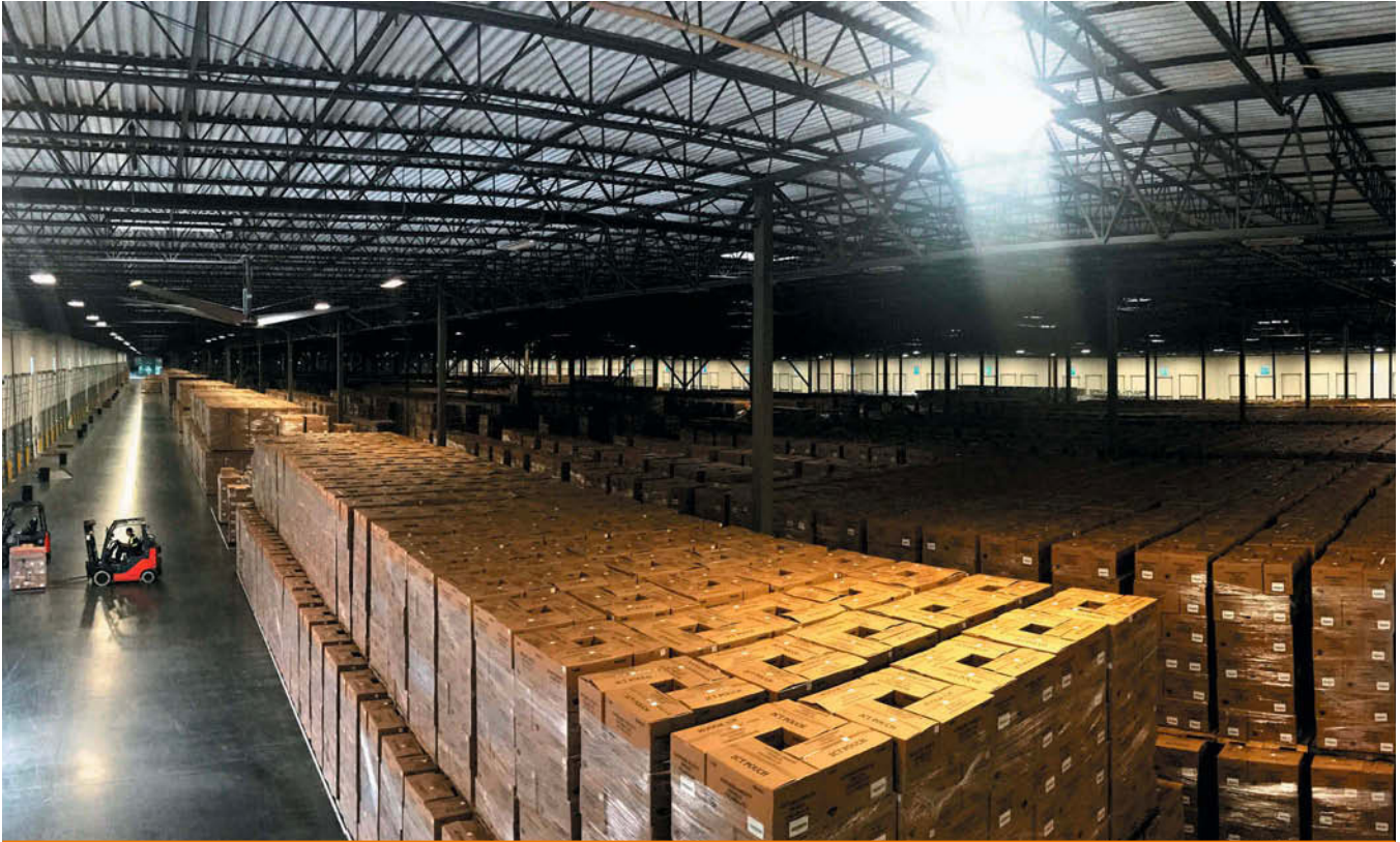
The Grimes Companies recently opened a 600,000 square-foot warehouse to handle domestic volumes as well as growth in Asian cargo.
