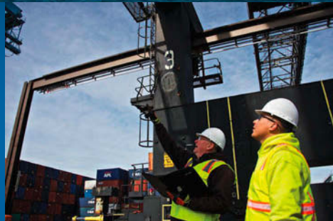
Crane demolition, Port Elizabeth, NJ
