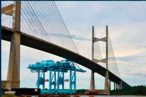
Crane relocation, Jacksonville, FL
