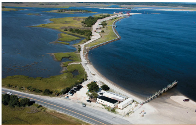
Aerial view of Mile Point.
