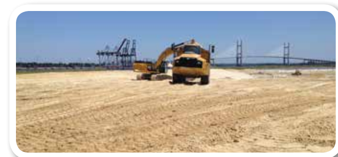
A dredge material operation in progress at Cell C
