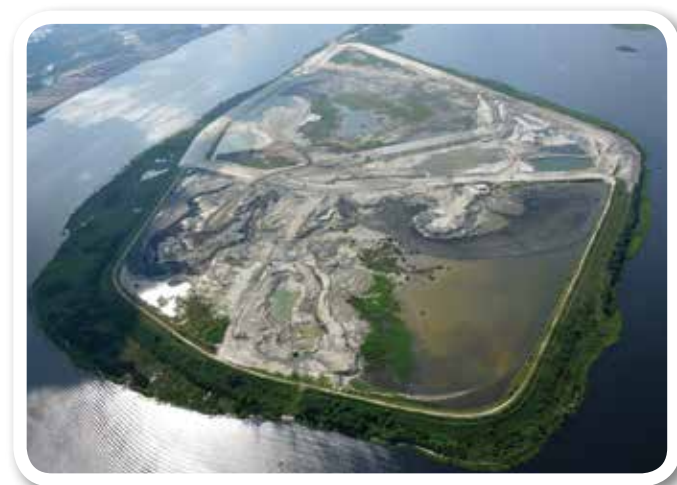
Aerial view of the Bartram Island Dredge Disposal facility, where storage capacity has been expanded
