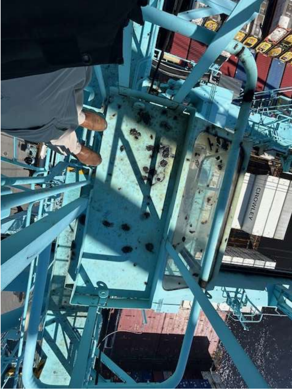
Photo Gallery Jaxport Cranes 10486-10487 Roofs
