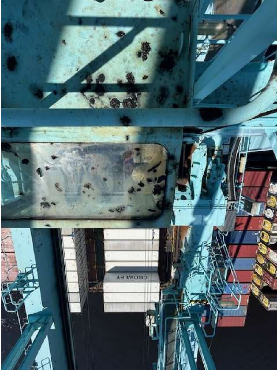
Photo Gallery Jaxport Cranes 10486-10487 Roofs
