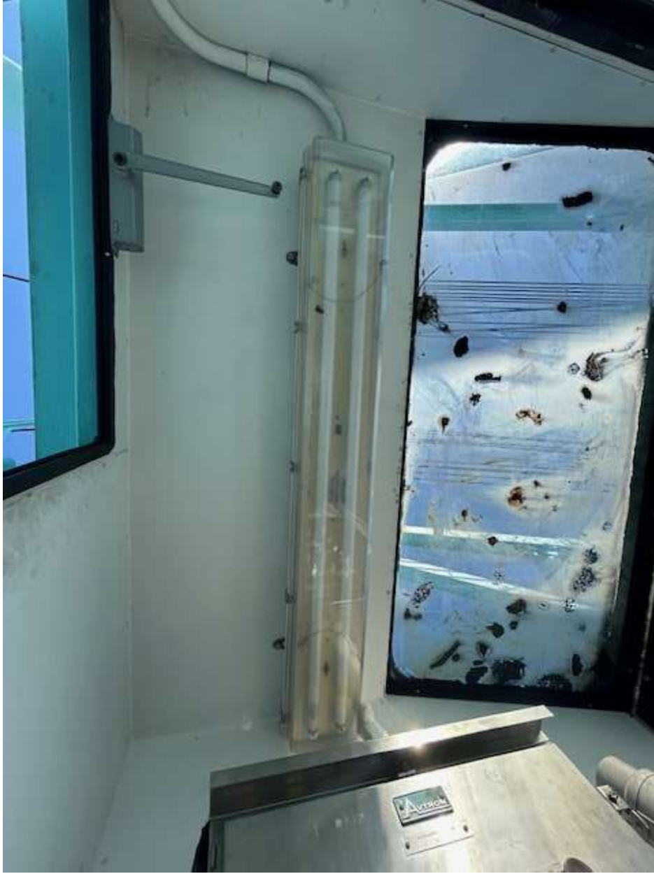
Photo Gallery Jaxport Cranes 10486-10487 Roofs
