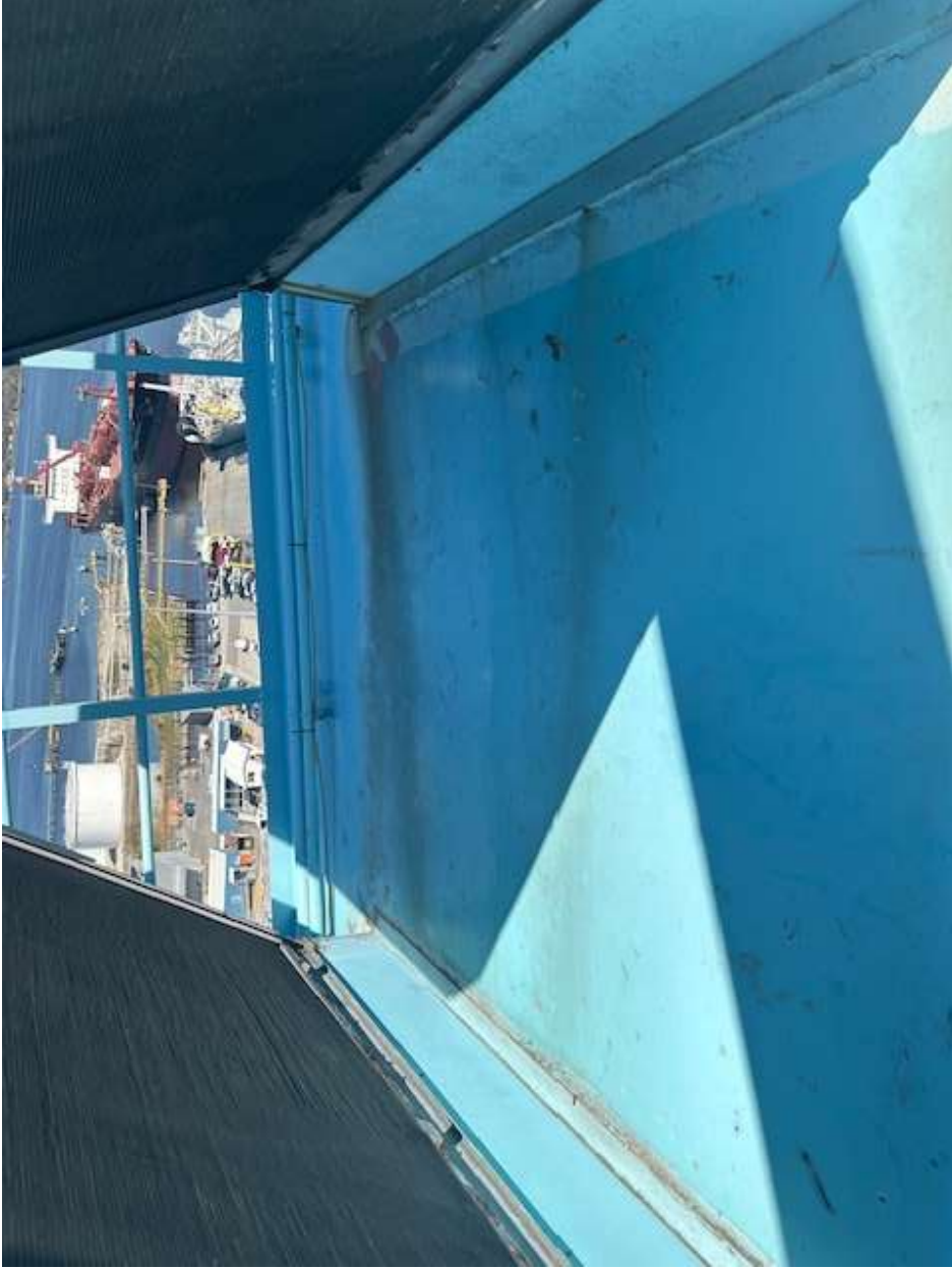
Photo Gallery Jaxport Cranes 10486-10487 Roofs
