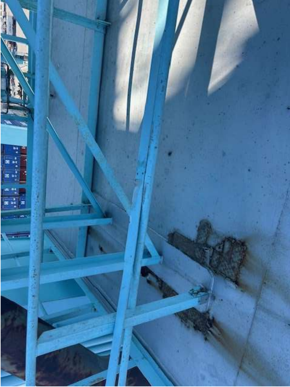
Photo Gallery Jaxport Cranes 10486-10487 Roofs
