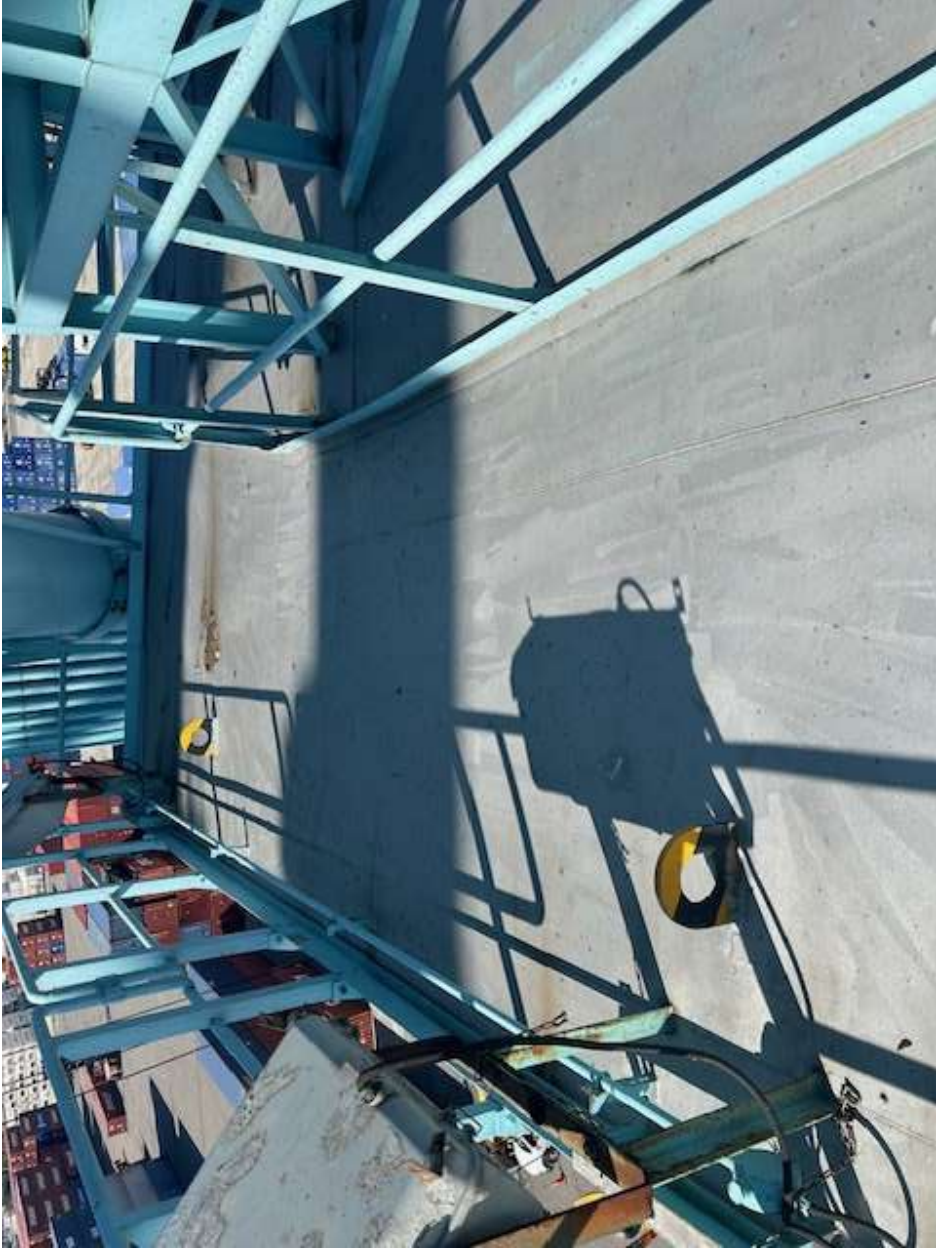
Photo Gallery Jaxport Cranes 10486-10487 Roofs
