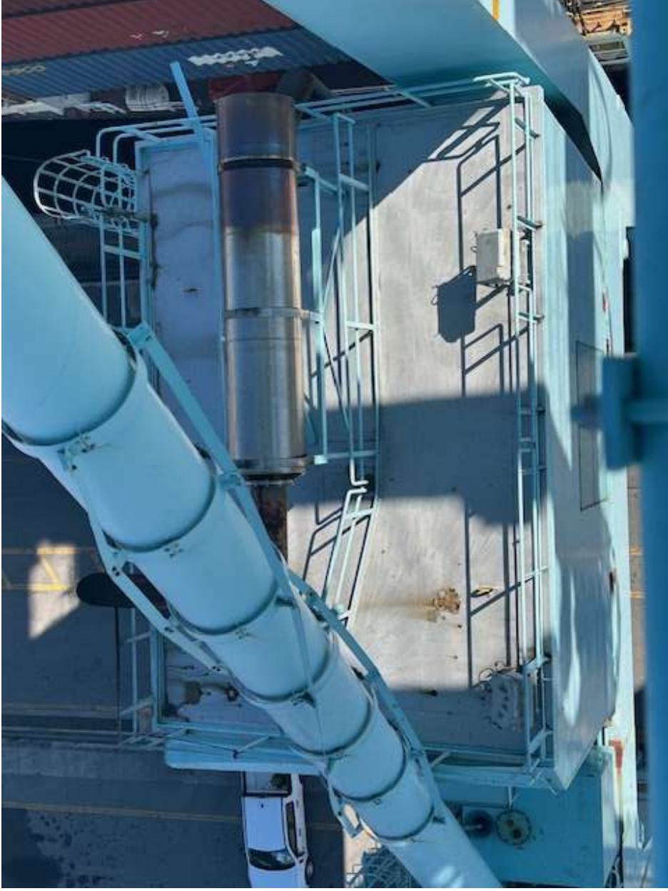
Photo Gallery Jaxport Cranes 10486-10487 Roofs
