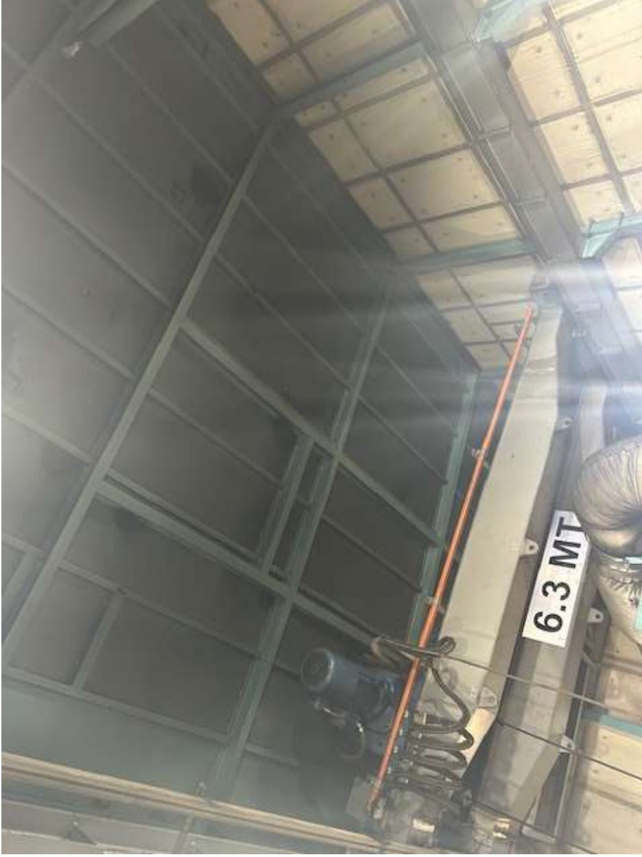
Photo Gallery Jaxport Cranes 10486-10487 Roofs
