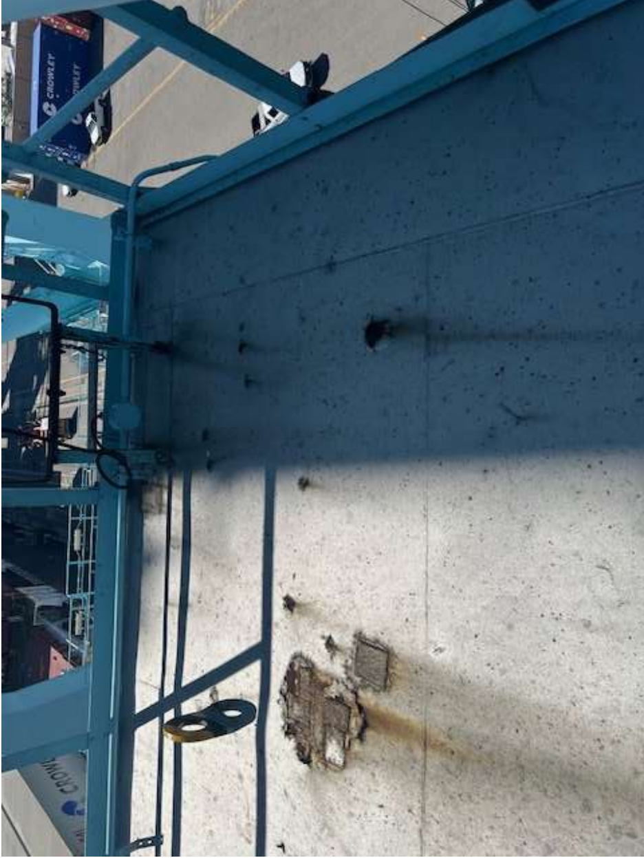
Photo Gallery Jaxport Cranes 10486-10487 Roofs
