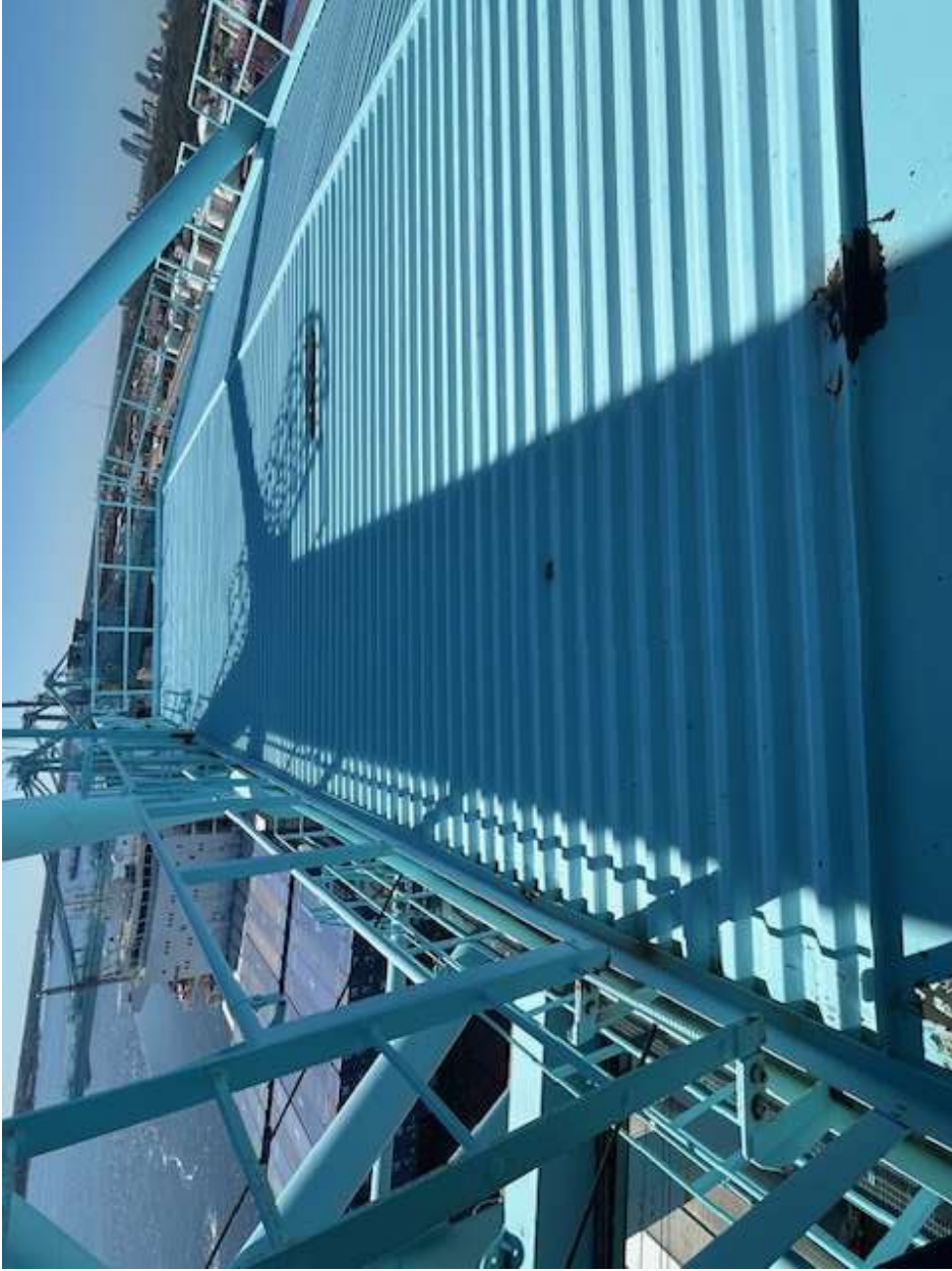
Photo Gallery Jaxport Cranes 10486-10487 Roofs
