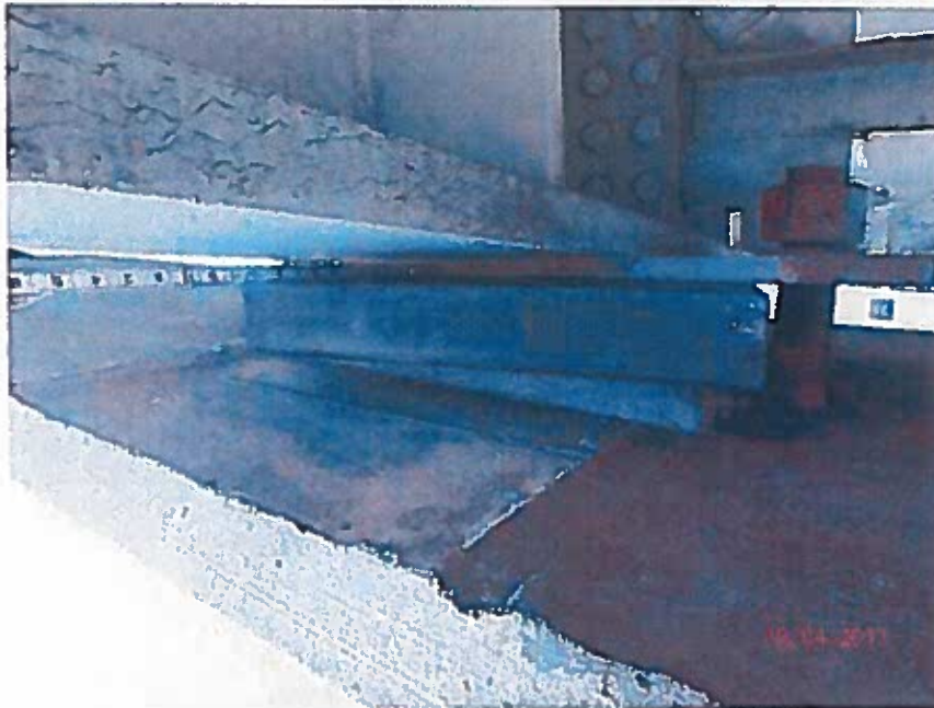
Photo 1: Bearing 9-2 Walking Out from Under Sole Plate
