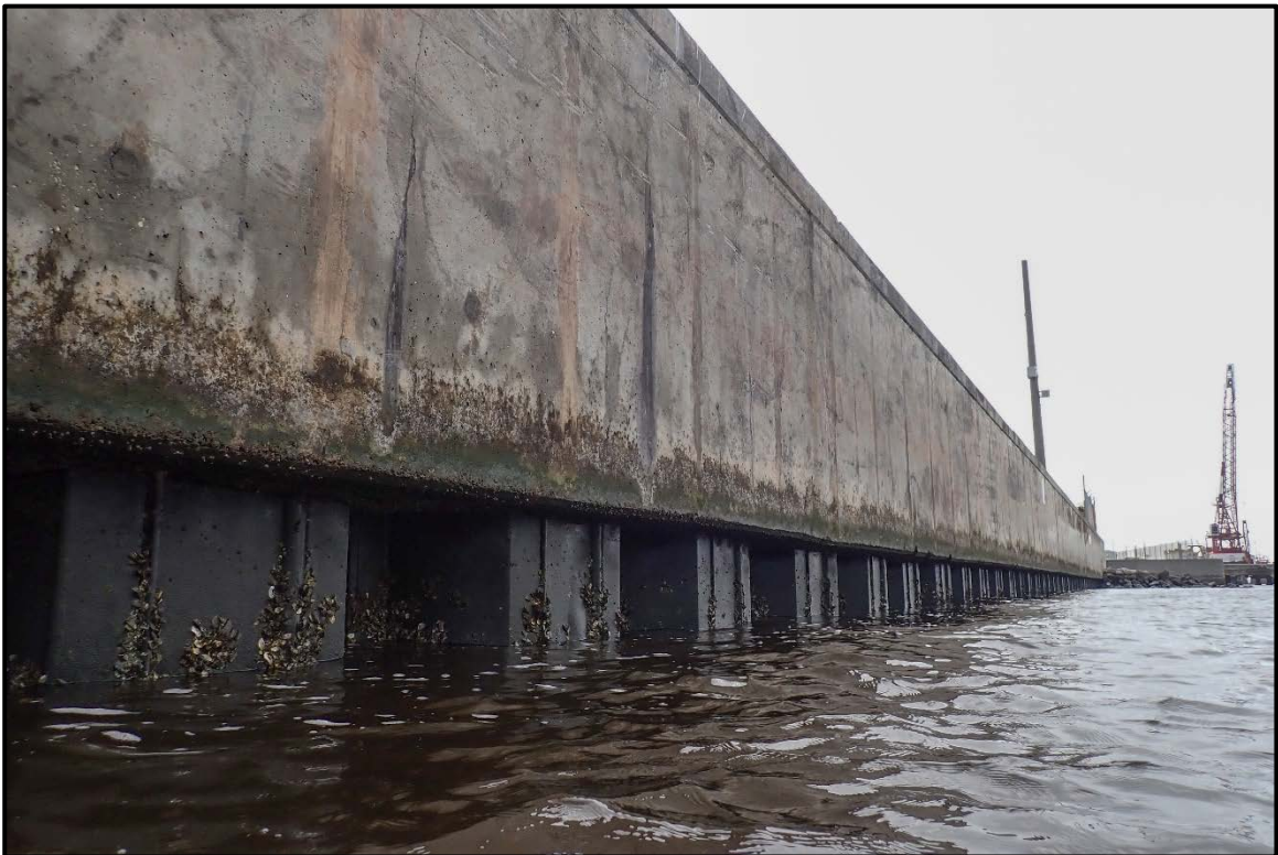
PHOTO 2-4 Typical view of bulkhead wall, looking south.
