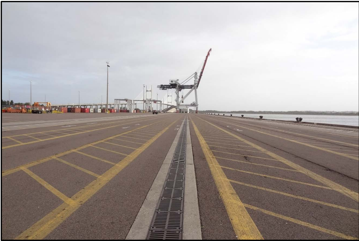
PHOTO 2-3 Topside view of Berth 17, looking south.
