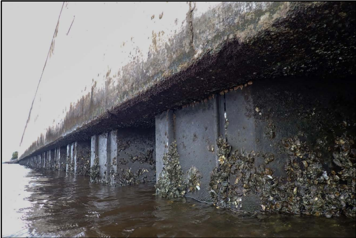
PHOTO 2-8 Bulkhead wall with intact epoxy coating.
