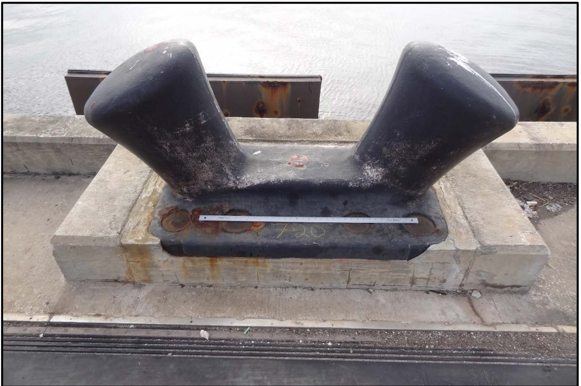
PHOTO 2-6 Typical 150-ton double-bit bollard.
