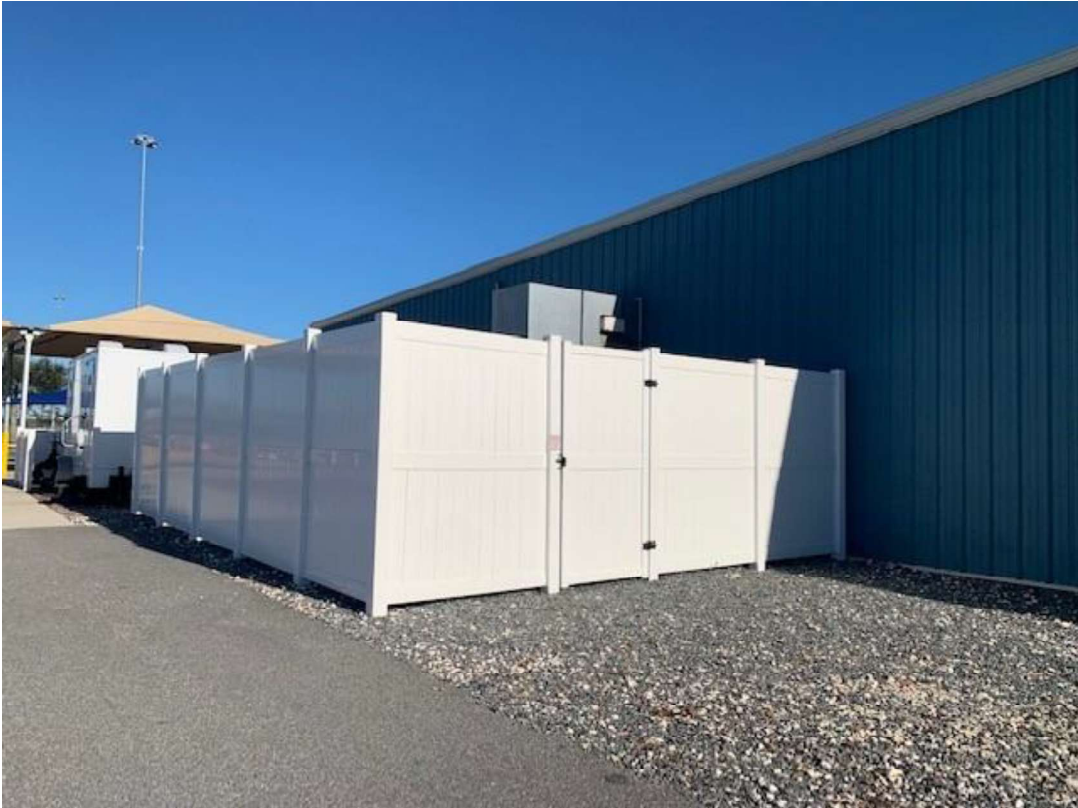
8' Tall Perimeter Fence with 4' Wide Entrance Gate
