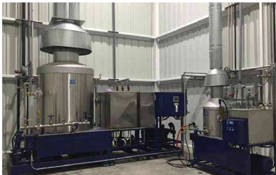
Single pass high pressure kosher washer system.
